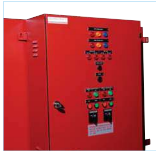
Sprinkler Pump Control Panel
