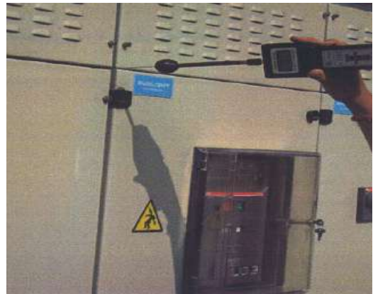
4.2d IP 4X in progress
