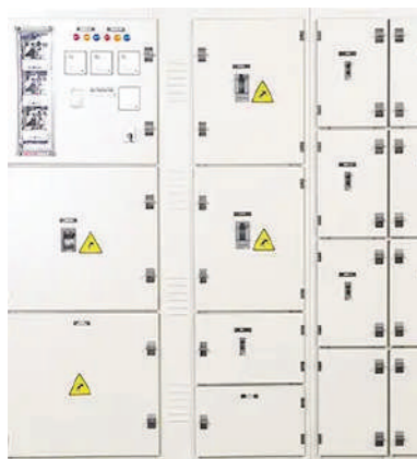
Sub Distribution Board
