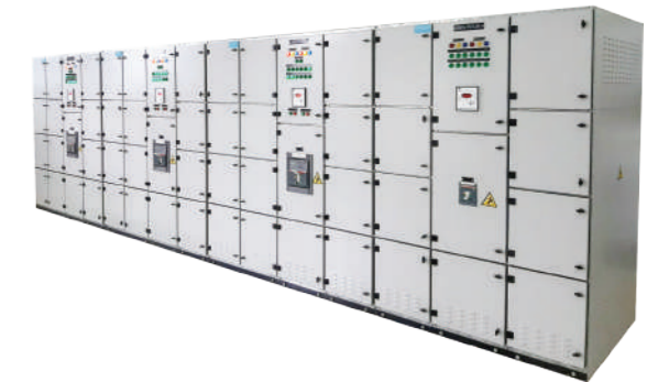
Power Factor Improvement Panel
